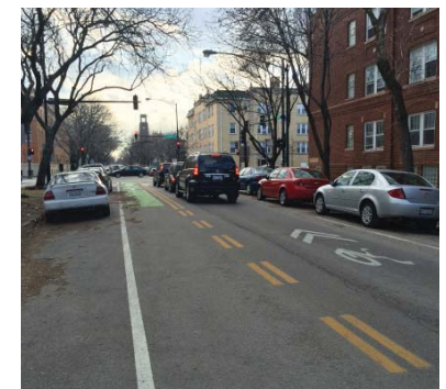
DASHED YELLOW LINES Help drivers and cyclists understand the appropriate lane position.
