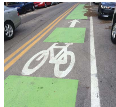
GREEN PAINT May be used near intersections to increase visibility of the contraflow bike lane.
