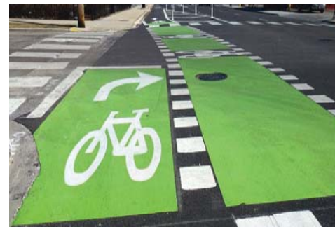
TWO STAGE TURN QUEUE BOX WITH BIKE LANE On streets with bike lanes, install turn queue box between the bike lane and curb.
