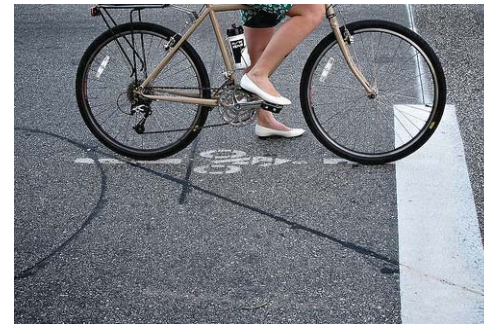
LOOP DETECTION Allows cyclists to trigger a signal without needing to push a button.
