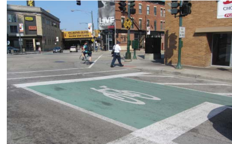
BIKE BOX Use at signalized intersections and place between the crosswalk and stop bar.
