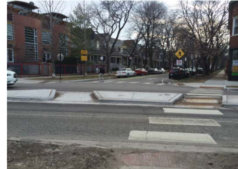
MEDIAN REFUGE ISLANDS Help both cyclists and pedestrians cross streets with high traffic volume.
