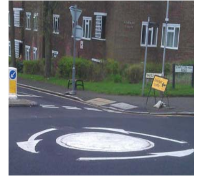
PAINTED MINI ROUNDABOUTS May be used prior to permanent installation, though they are not as effective. Photo credit: http://www.lbc.co.uk/
