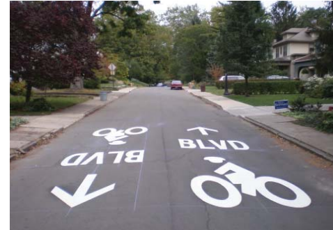
NEIGHBORHOOD GREENWAYS PAVEMENT MARKING Use along Neighborhood Greenways, spaced 250 feet apart. Photo credit: http://www.columbusunderground.com/
