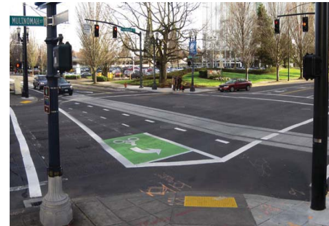
TWO STAGE TURN QUEUE BOX Can be used at offset intersections on streets with high traffic volumes. Photo credit: NACTO
