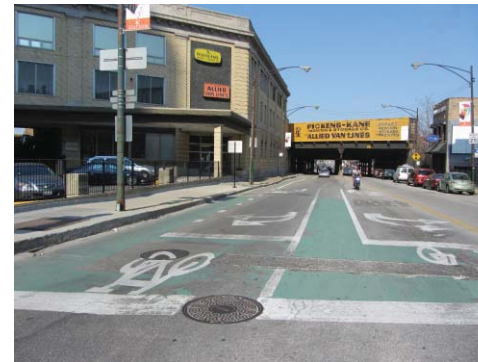
NEIGHBORHOOD GREENWAYS PAVEMENT MARKING WITH TURN ARROW Are used where Neighborhood Greenways are offset, jog, or where two Neighborhood Greenways intersect. Photo credit: J. Maus
