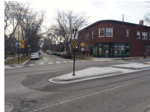
MEDIAN REFUGE ISLANDS May also be used to prohibit car turning movements onto Neighborhood Greenways.
