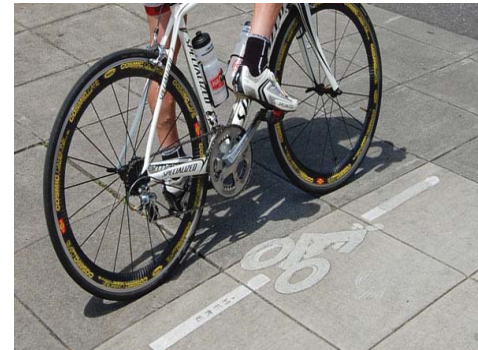
BICYCLE LOOP DETECTOR Enables cyclists to trigger signals at lights without needing to dismount. Photo credit: NACTO
