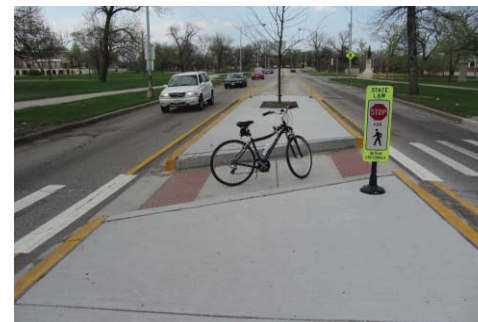
CUT-THROUGHS Should be designed to accommodate cyclists, people in wheelchairs, and strollers.
