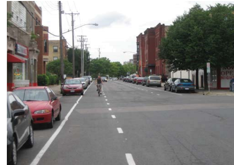
ADVISORY BIKE LANES Advisory bike lanes give cyclists a defined space to travel in mixing zones. Image credit from top to bottom: streets.mn (top), bikemiami.org (middle), Steve Clark (bottom)
