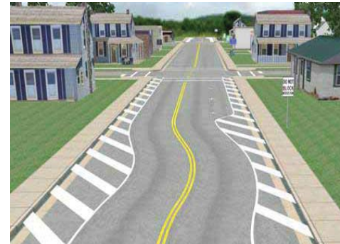
TEMPORARY CHICANES Temporary installations may be used prior to permanent installation. Temporary installations can be created through paint, temporary curbs, giant flower pots, or other creative uses. Photo credit: FHWA
