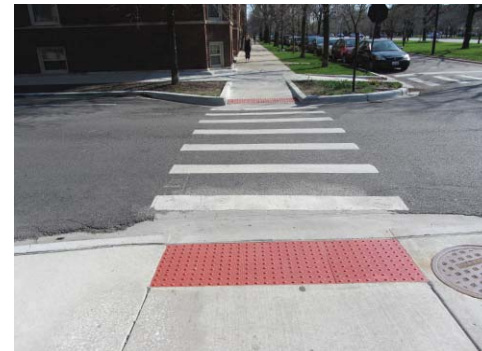
CURB RAMPS AND TACTILE PADS Should be installed at culs de sac along the Neighborhood Greenways network. These facilities help cyclists, wheelchair users, and people pushing strollers.
