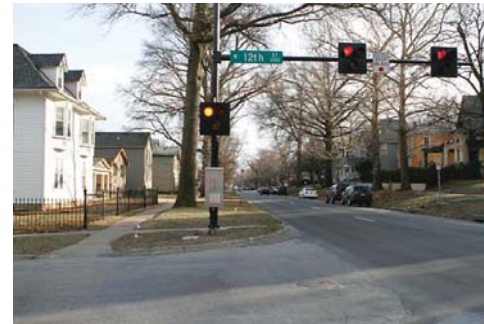
HAWK SIGNAL Use at uncontrolled crossings where Neighborhood Greenways intersect streets with high traffic volumes. Photo credit: C. Bronson.
