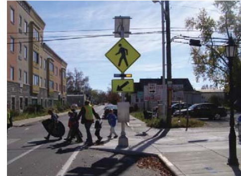
RECTANGULAR RAPID FLASHING BEACON Use at uncontrolled crossings where Neighborhood Greenways intersect streets with high traffic volumes. Image credit: bloomington.in.gov
