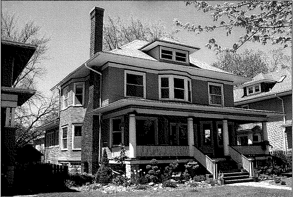
South and East Elevations
