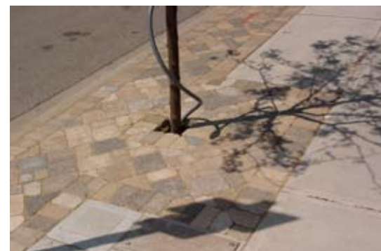
Electrical With Pavers
