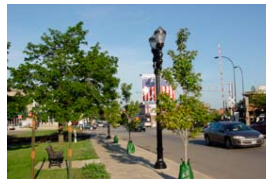
Pedestrian Sidewalk Light
