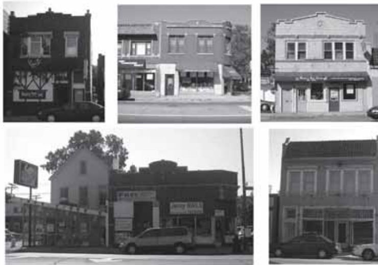
Examples of the existing scale of buildings along the corridor.
