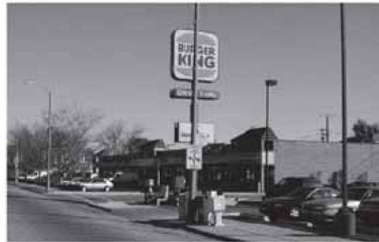
When auto-oriented properties such as this strip mall get redeveloped, mid-story buildings should be constructed at the sidewalk.
