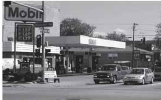
Existing gas station has no buffer.
