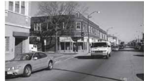
Some areas of Subarea 6 have intact streetwalls and need some renovations only.
