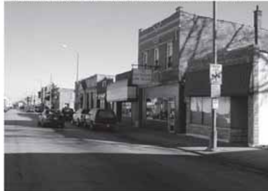
Update facades while preserving historic features.
