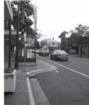
Bulb-outs drastically reduce amount of pavement to cross and allow space for pedestrian amenities.
