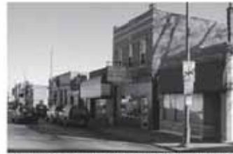
Storefronts at the sidewalk edge provide a rewarding pedestrian experi-
