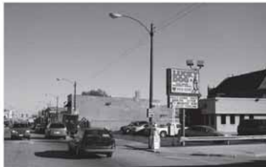
Some areas of Subarea 6 have eroded streetwalls and need major redevelopment.
