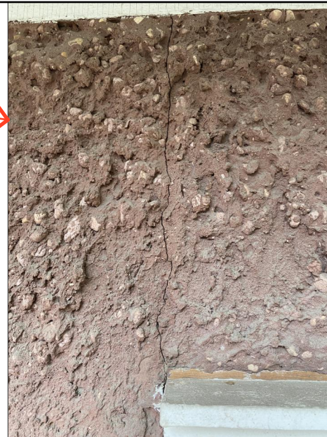
12. STUCCO CRACK 2
