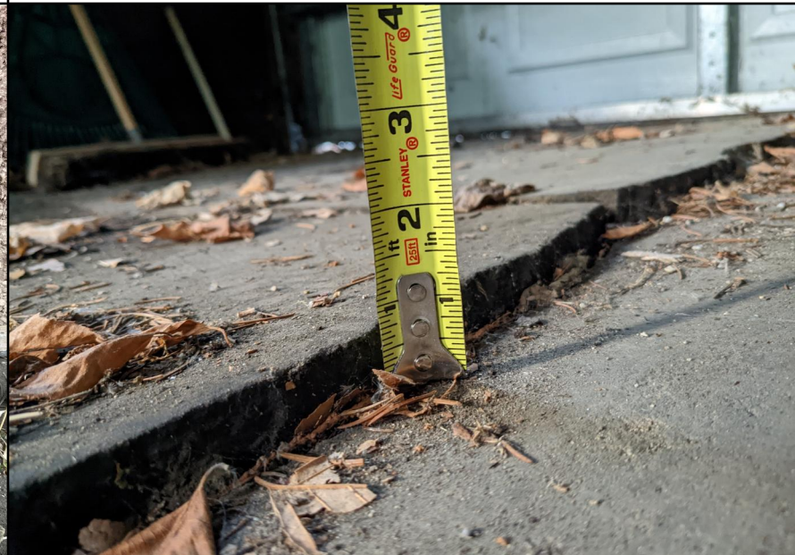
8. SLAB CRACK
