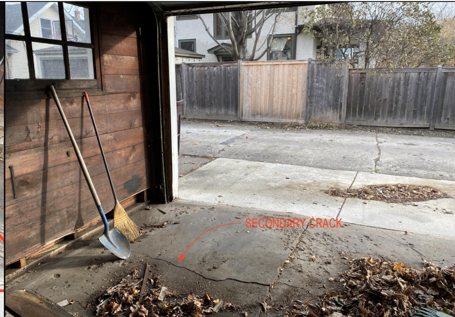
6. SLAB NORTH-EAST CORNER INTERIOR
